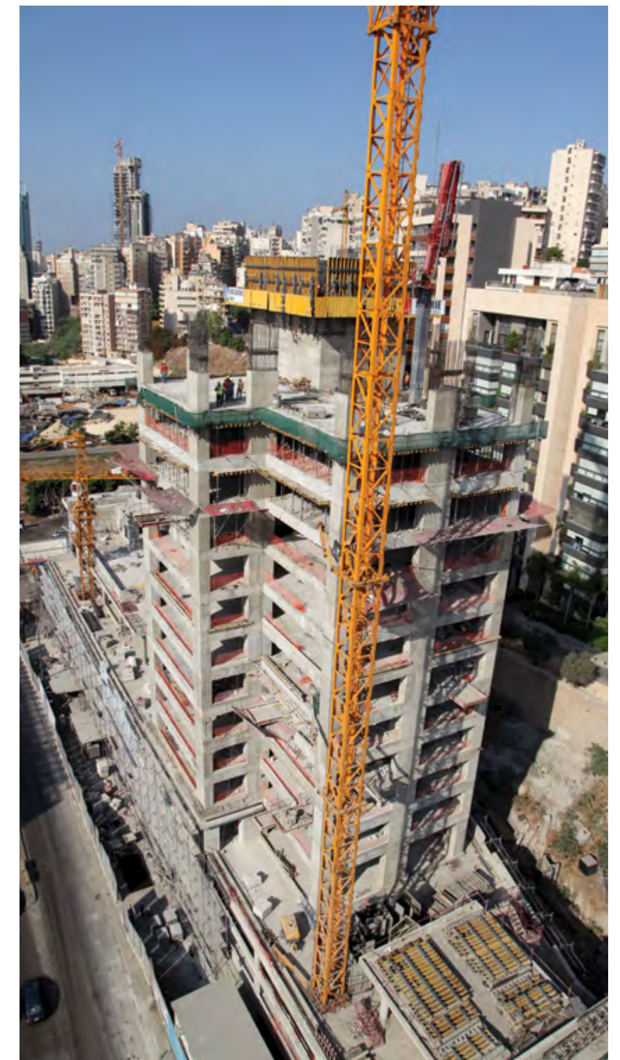
CRANES AND CONCRETE-PLACING BOOM ON SITE
