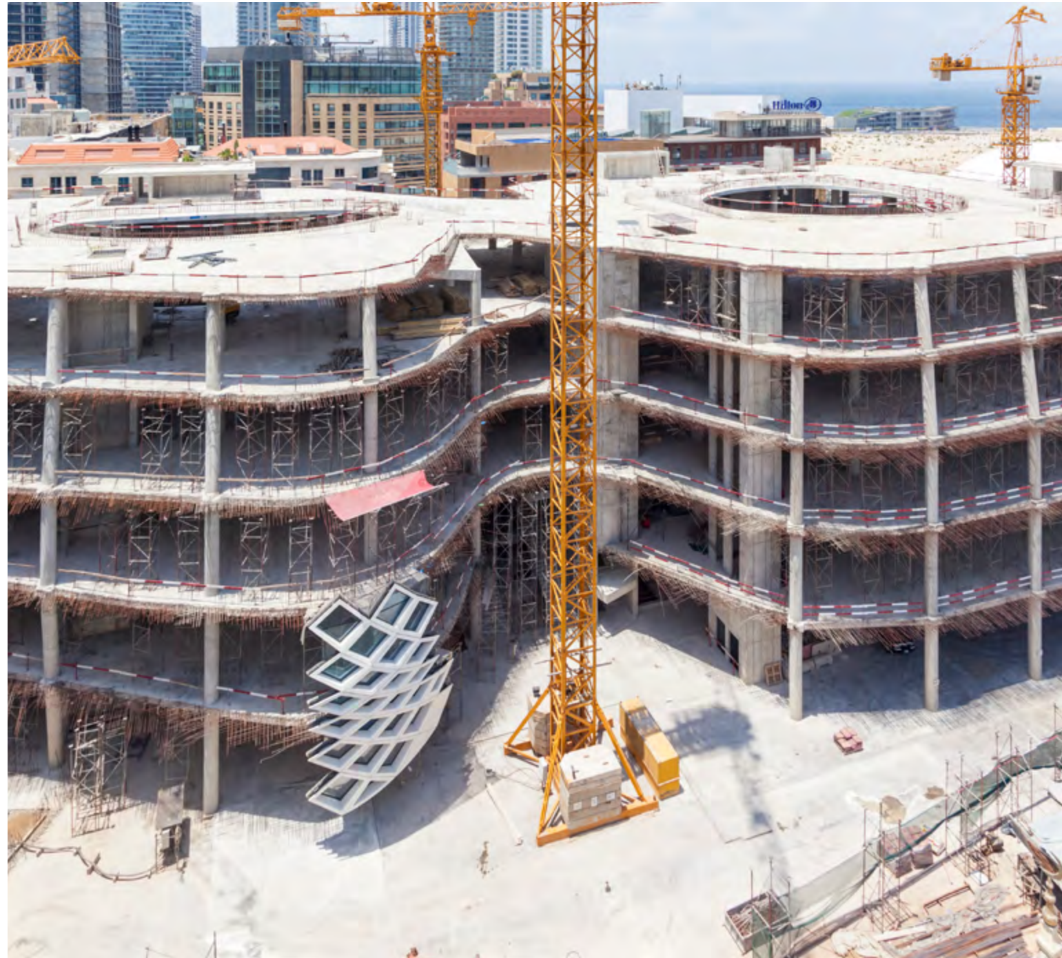
THE DISTINCTIVE FAÇADE WITH THE MOCK-UP OF G.R.C. ALUMINUM AND GLAZING
