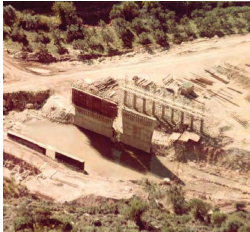
SHUTTERING AND EXECUTING PIERS AND ABUTMENT BRIDGE
