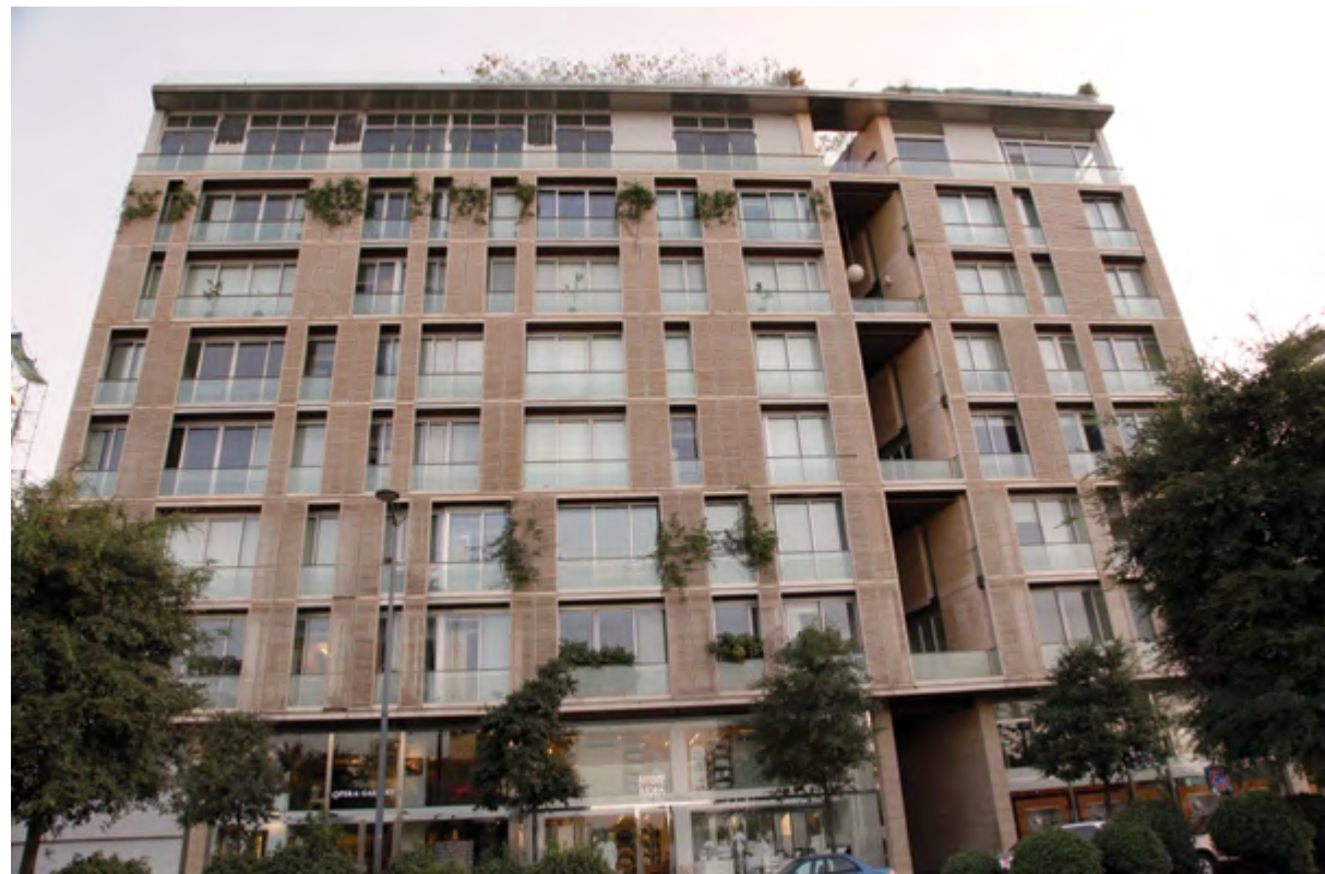
ELEVATION MIX OF STONE LOUVERS FIXED ON STAINLESS STEEL FRAMES AND STRIPS ALONG BUILDING PERIMETER, AND STAINLESS STEEL FALSE CEILING AT ROOF
