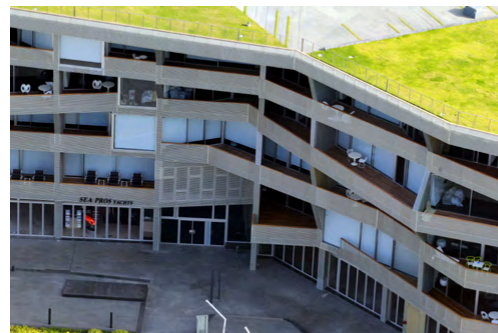
ZIGZAG BALCONIES WITH GALVANIZED ALUMINUM PERFORATED PANEL CLADDING
