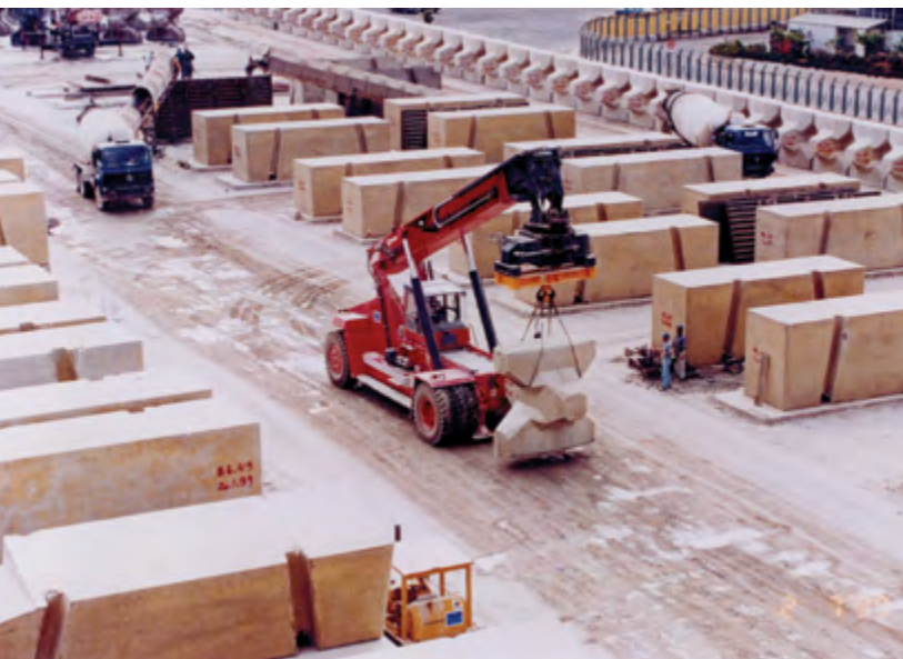
LIFTING ACCROPODE THROUGH THE CONCRETE BLOCKS STORAGE YARD
