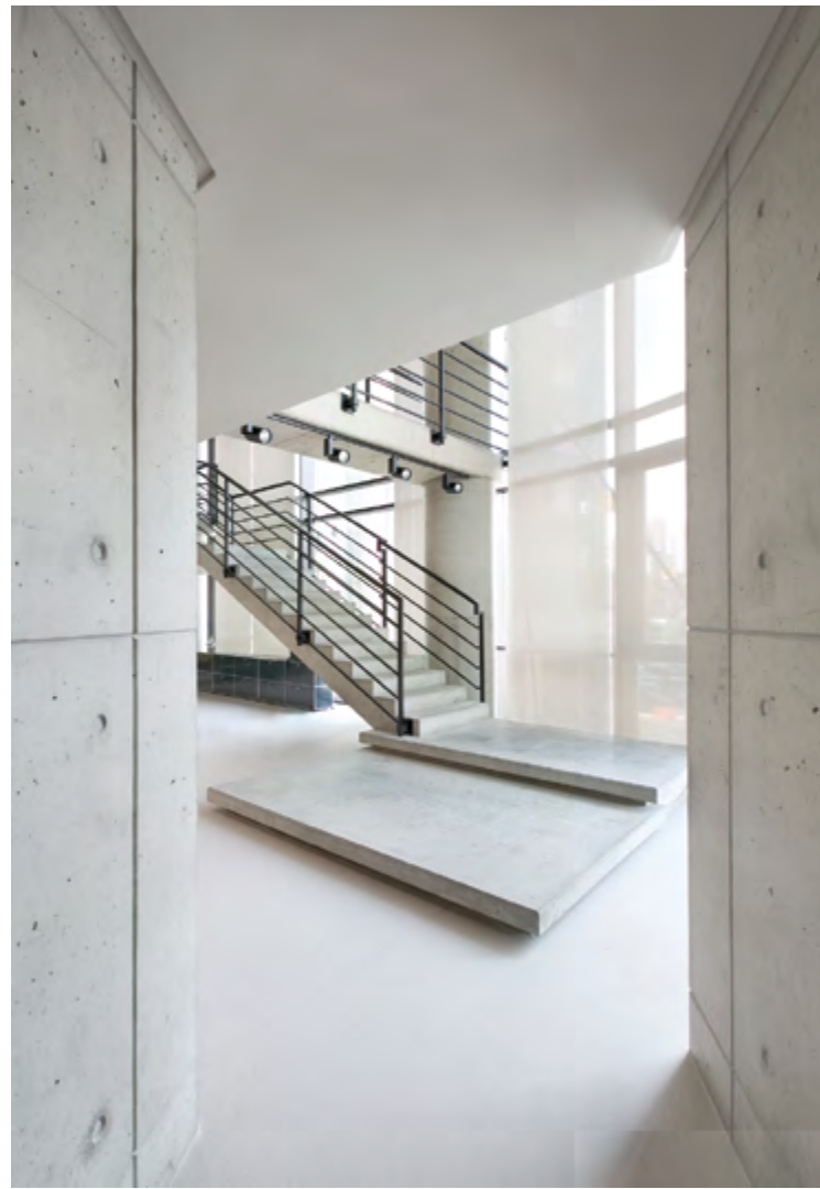
THE DETACHED CONCRETE STAIR WITH ITS CENTRAL LANDING AND BLACK METAL BALUSTRADE AND HANDRAIL LEADING ONTO THE MEZZANINE FLOOR
