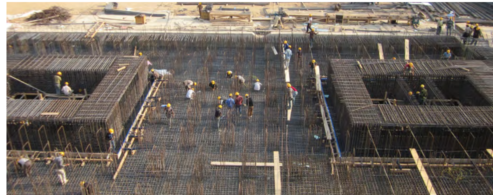
STEEL REINFORCEMENT FOR THE RAFT AND ELEVATOR PITS
