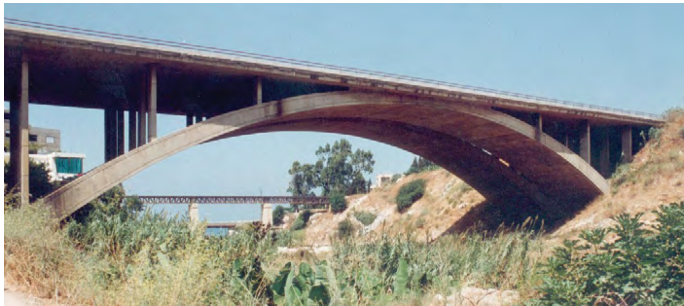
THE MAIN POST-TENSIONED ARCH
