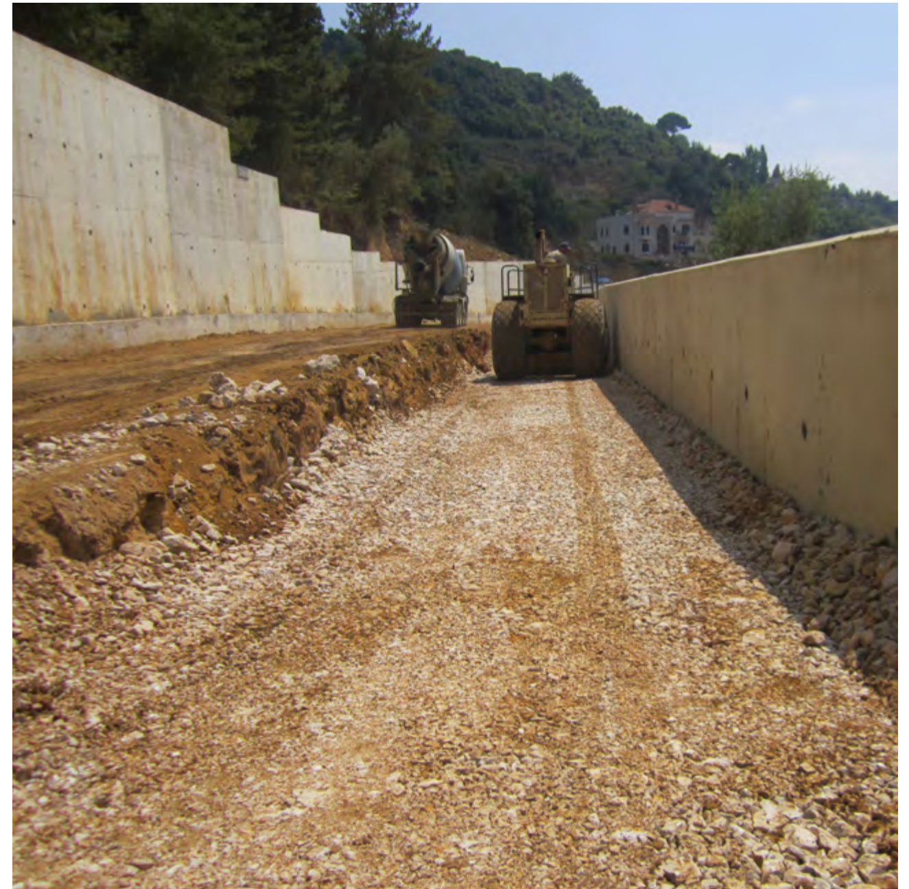
INSTALLATION OF BASE COURSE ADJACENT TO RETAINING WALLS
