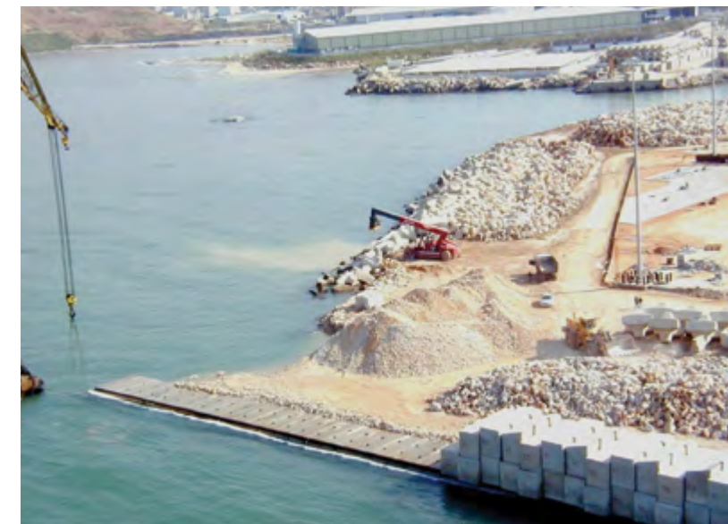
SLOPE-AND-SCOUR PROTECTION WORKS
