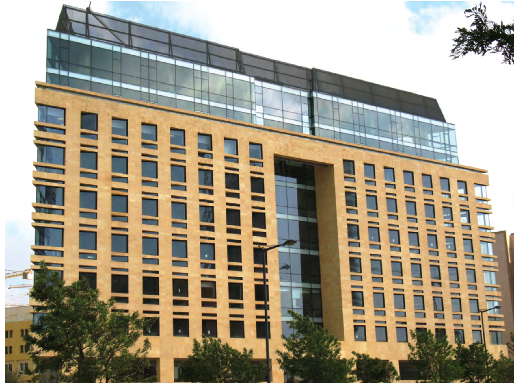
FAÇADE REFLECTING MIX BETWEEN ACOUSTIC LOUVERS, STONE, GLASS AND ALUMINUM CURTAIN WALL
