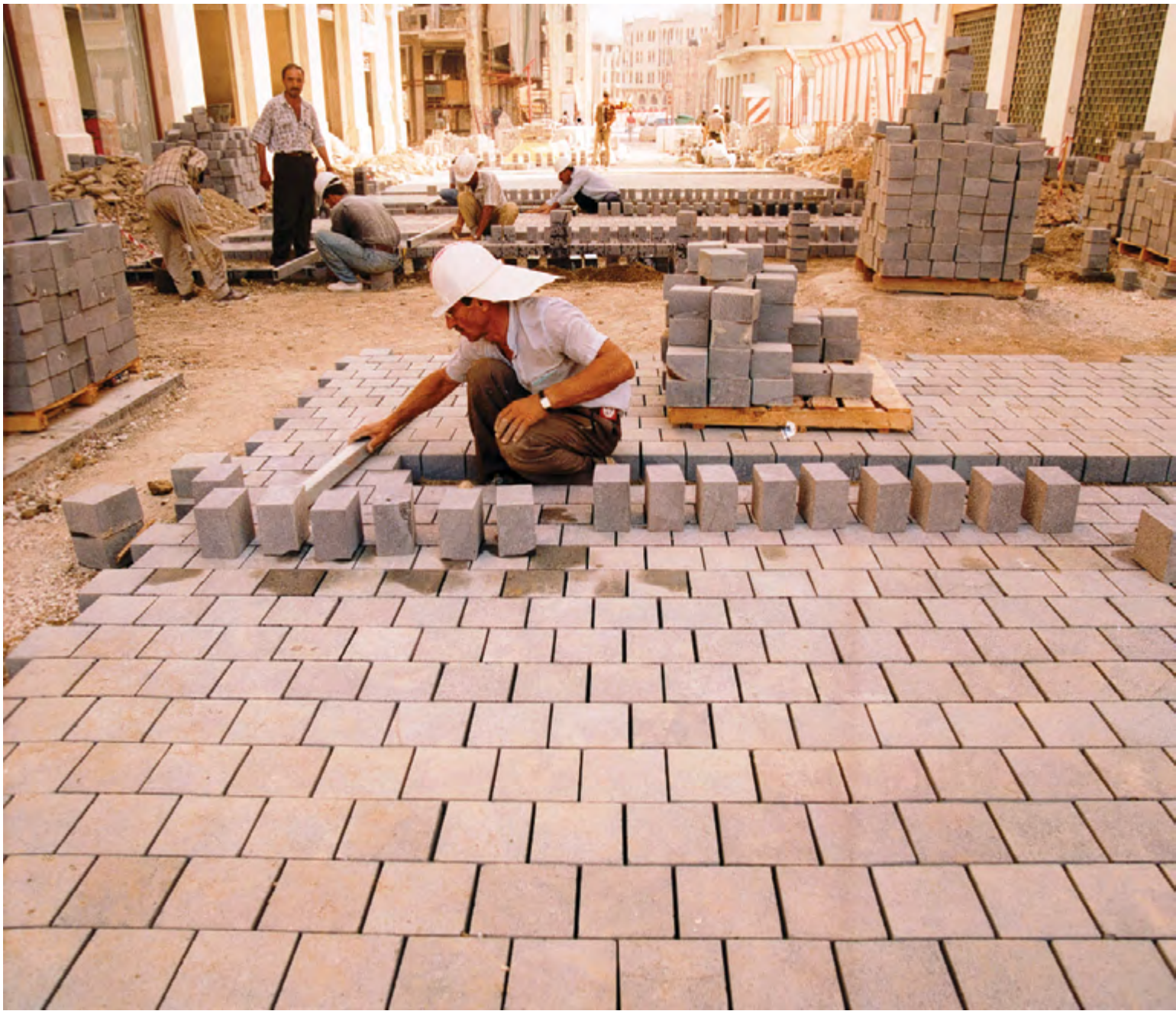
LAYING COBBLESTONE PAVEMENT
