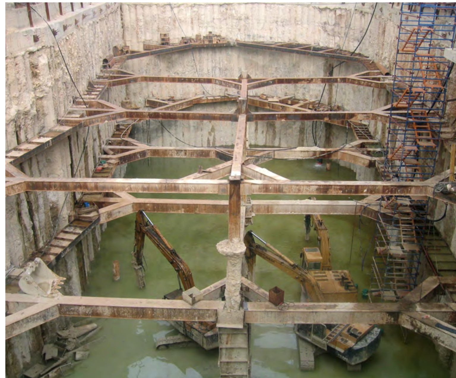
CROSS BRACING OF FOUNDATION WALLS
